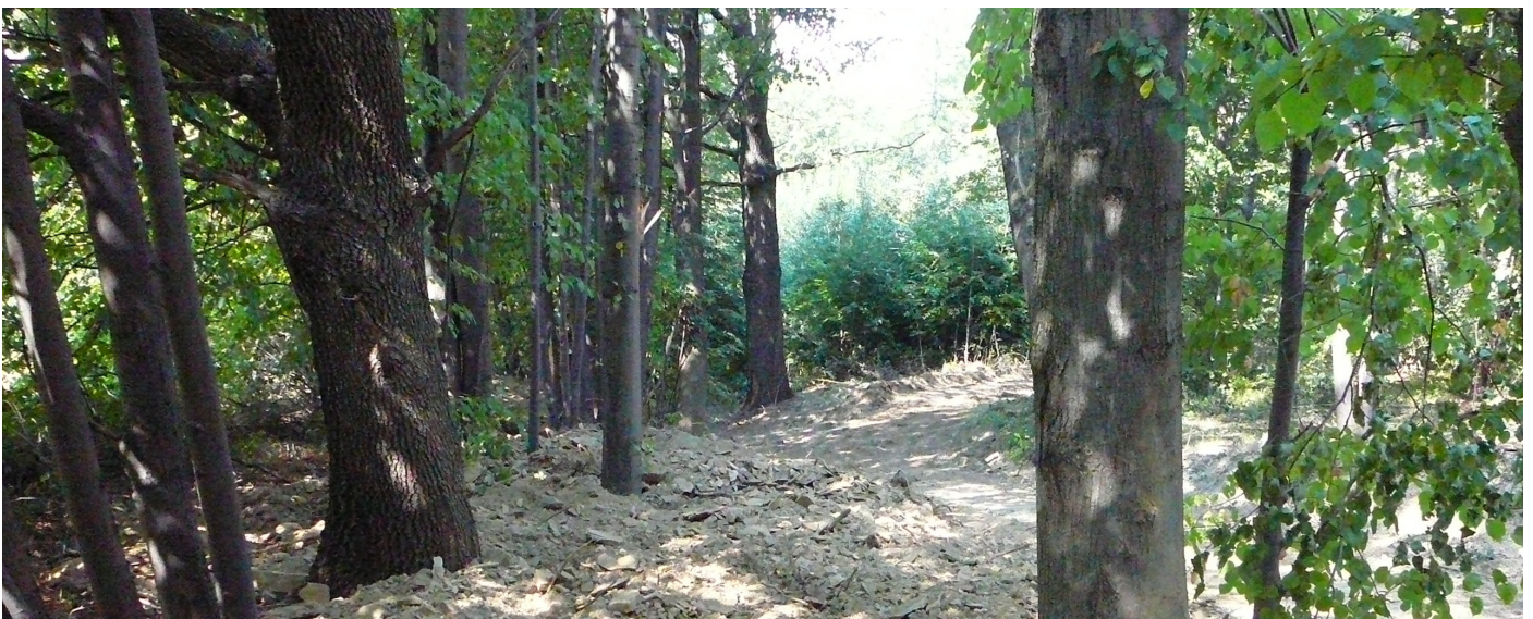
Trees buried during a new road construction .
